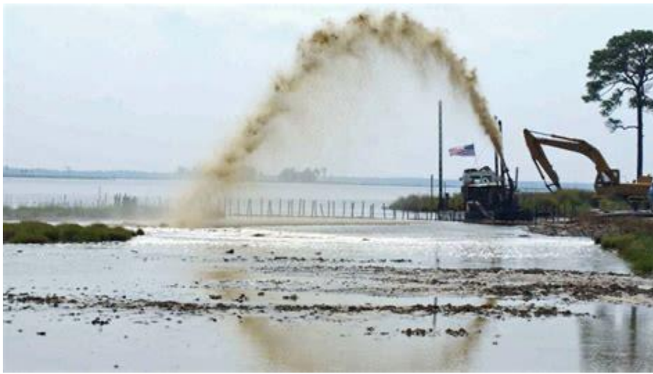
Thin layer placement of sediment on a coastal wetland
