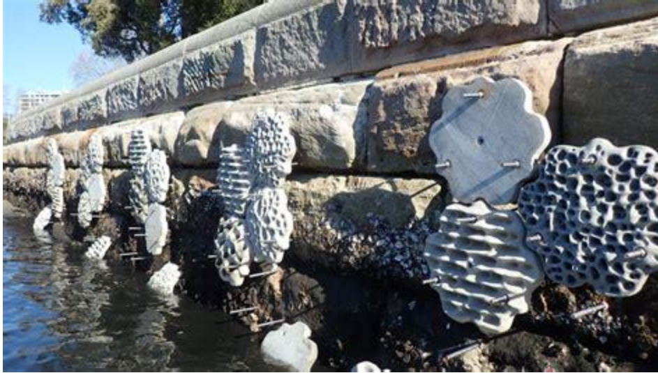
A living sea wall project in Australia
