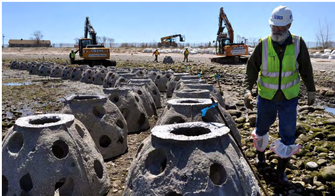
← Installation of Reef Balls
