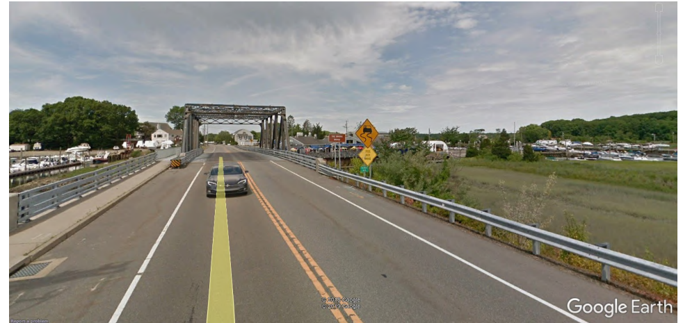
Figure 3-8: Portion of Boston Post Road located in the FEMA Special Flood Hazard Area that is inundated during the 100-yr recurrence interval flood.
