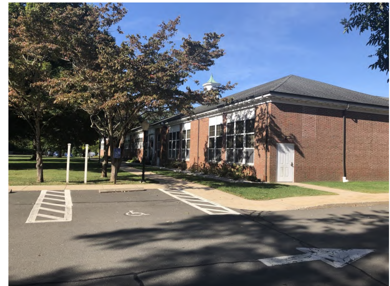
Image of Westbrook Town Hall at 866 Boston Post Road
