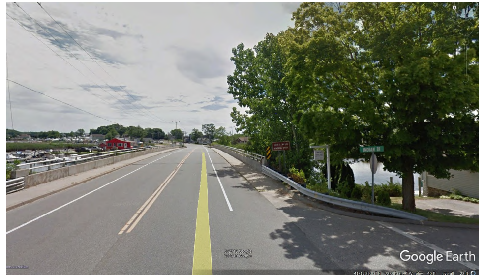
Figure 3-9: Portion of Boston Post Road located in the FEMA Special Flood Hazard Area that is inundated during the 100-yr recurrence interval flood.
